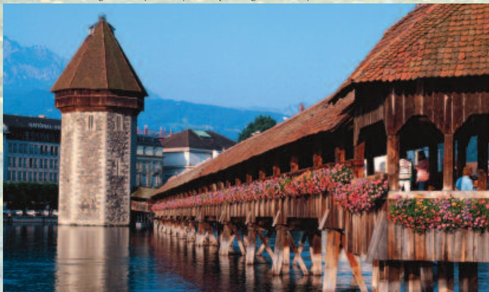
Alpine flowers adorn the railing of Lucerne's 14th-century Kapellbrücke (Chapel Bridge), Europe's oldest covered wooden bridge, which features famous paintings on its roof's interior.
