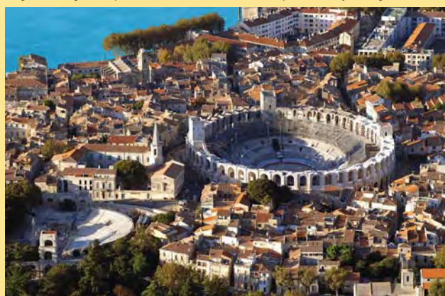
Arles' Romanesque architecture reflects its history as an important port of call on the Roman road from Italy to Spain.
